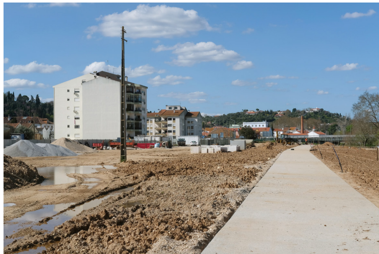
© António Ventura 2025 Figure 4 - Flecheiro riverside park in Tomar, working in progress 2023 -2024
