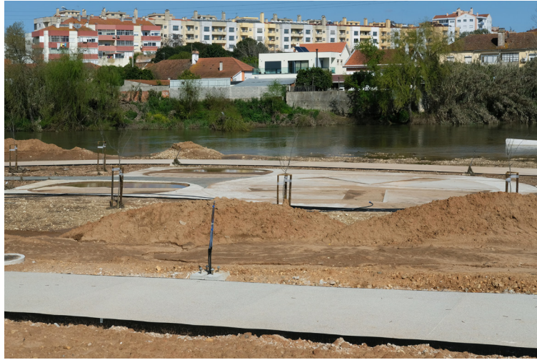
© António Ventura 2025 Figure 3 - Flecheiro riverside park in Tomar, working in progress 2023 -2024
